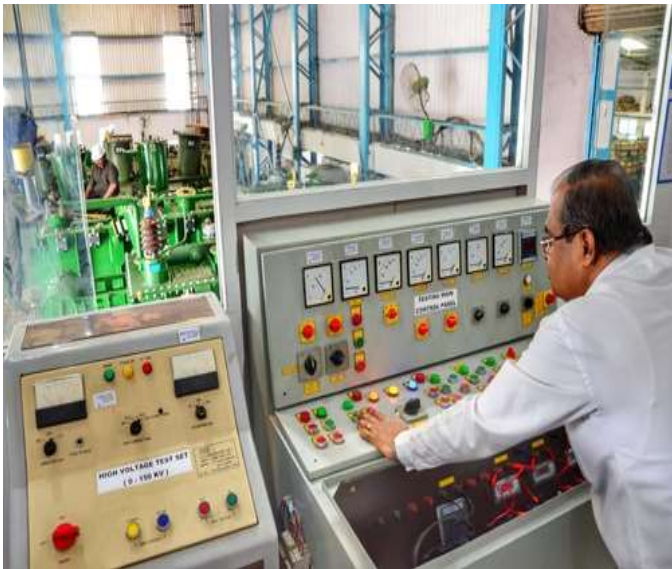
High Voltage Transformer Testing
